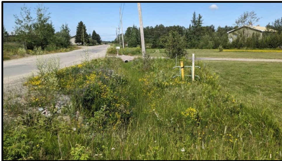
Image 21. Photograph 5639, looking west along the drainage ditch on the north side of Oil Tank Road.
